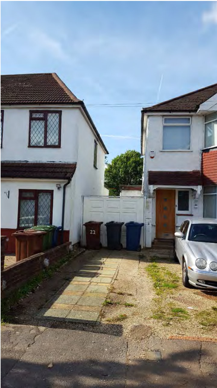
View of gap between No.22 and No. 24
