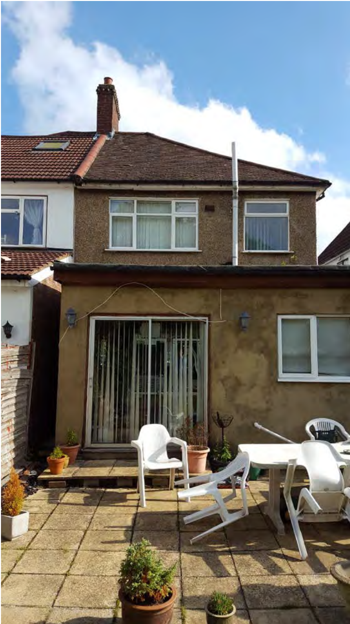
View of rear of dwelling
